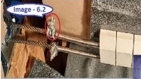
Steel wire rope clip M5 should face opposite to the pulley as shown in right Image.
